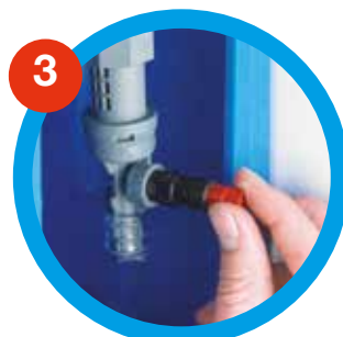
Screw it into the stub
